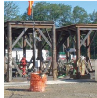
Well Head Cages for Infield Drilling
