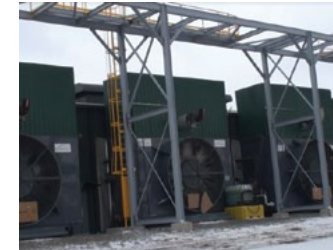
Platforms, Walkways and Stairs
